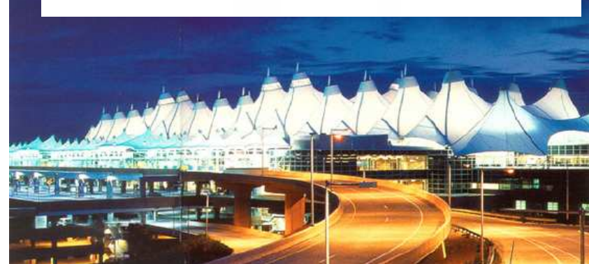
Denver International Airport, USA
